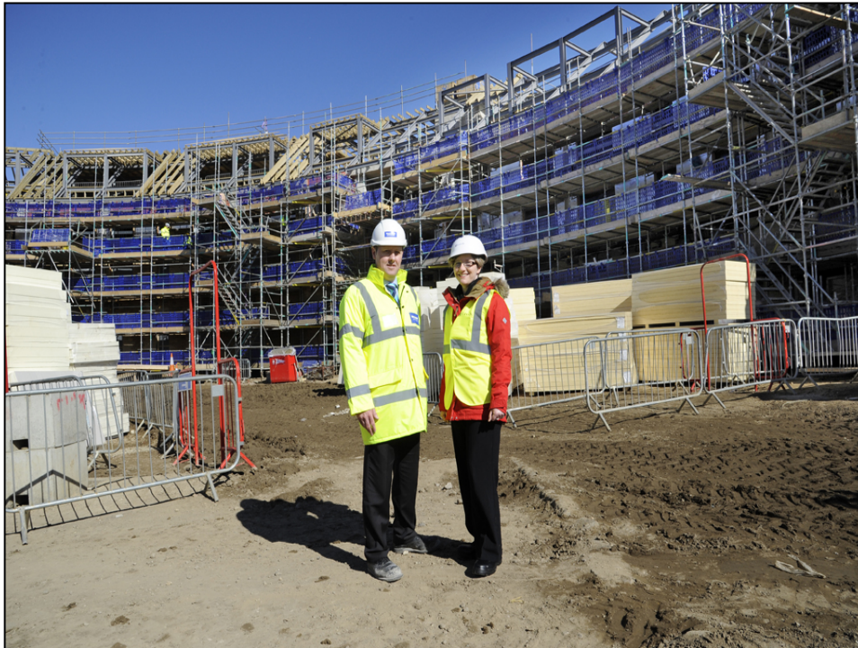
Wharfedale View, Yeadon - extra care development replacing outdated sheltered stock.
